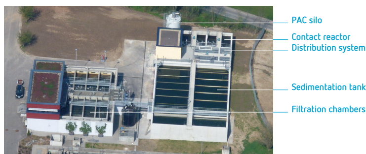
Figure 2 Aerial photo of the adsorption stage and filtration plant (photo: Rolf Mugele)
